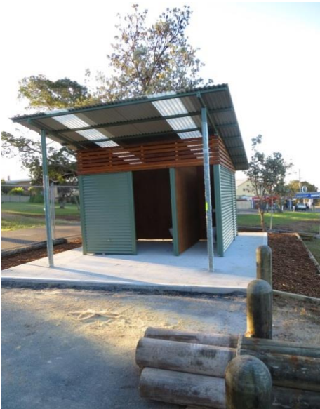
Hall Reserve toilet block under construction.
