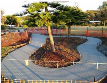
The Bike track under construction
